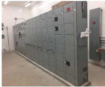
**Photos:** *Prefabricated Blower Electrical Building and Switchgear*
